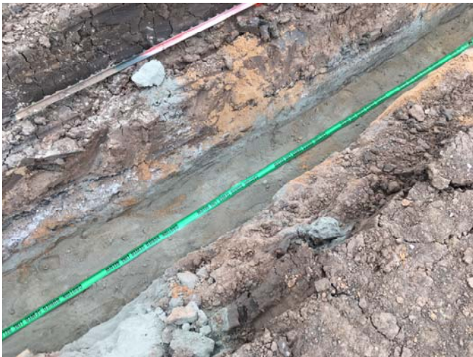
3. Site sanitary piping
