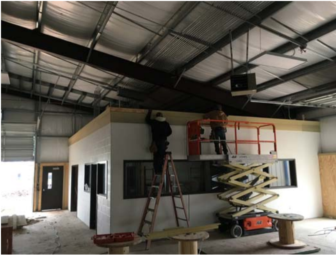
9. Hardi trim at classroom
