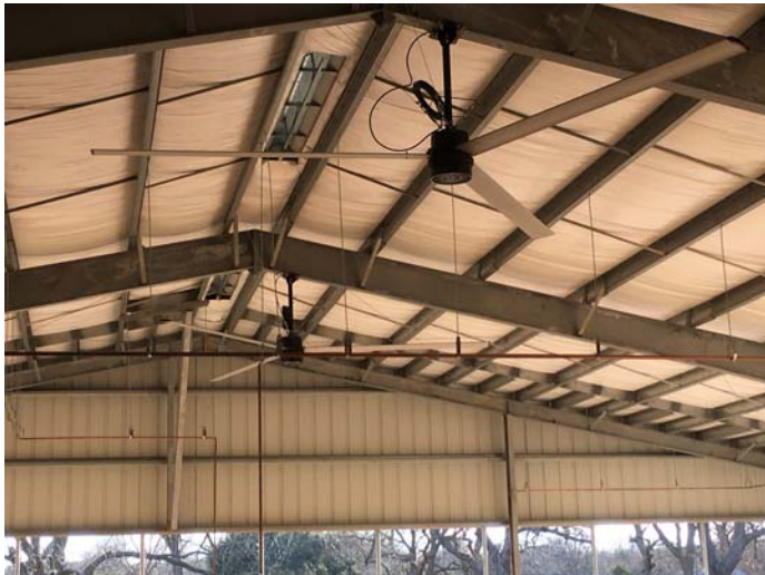
1. HVLS fan installation
