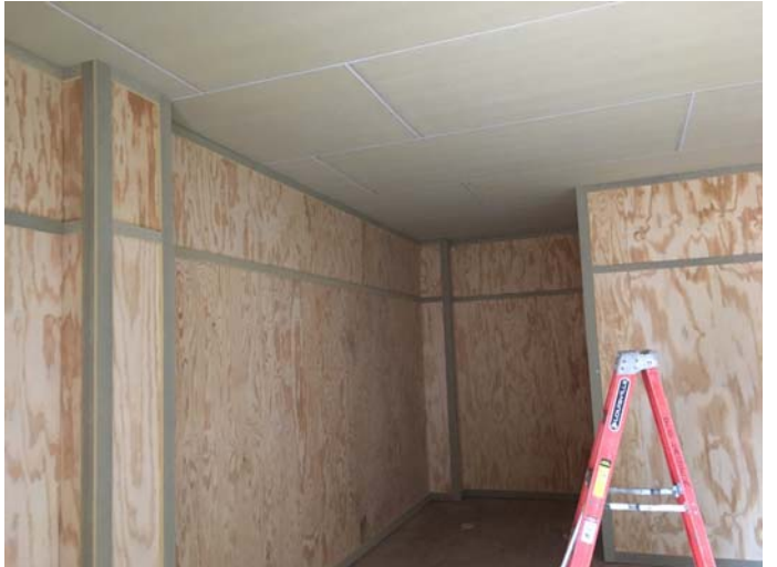
6. Interior plywood and trim at Storage Pens
